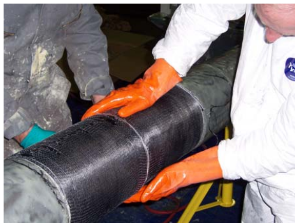
Figure 16 – Installation of composite repair
