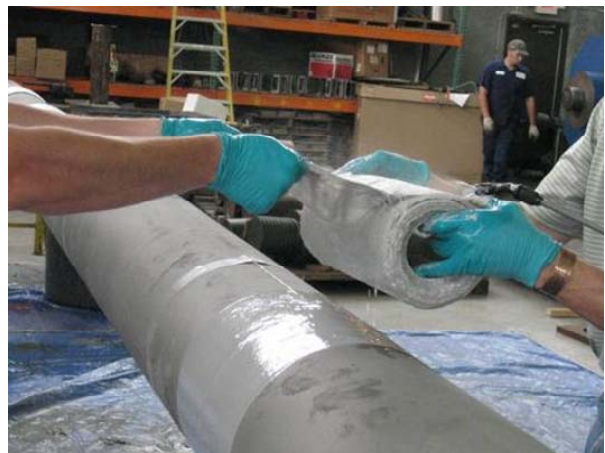
Figure 5 – Installation of composite systems that participated in dent repair program
