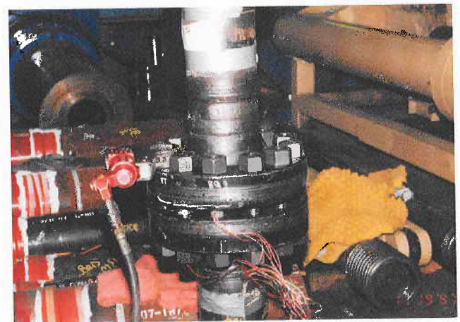
Figure 2 Flange assembly during makeup
