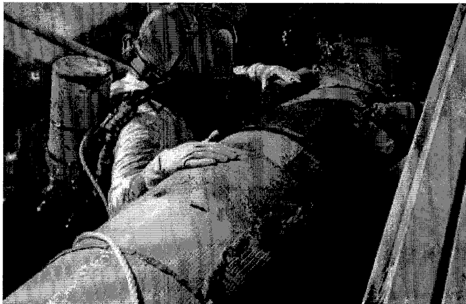
Figure 5 Repair of offshore pipeline using APPW
