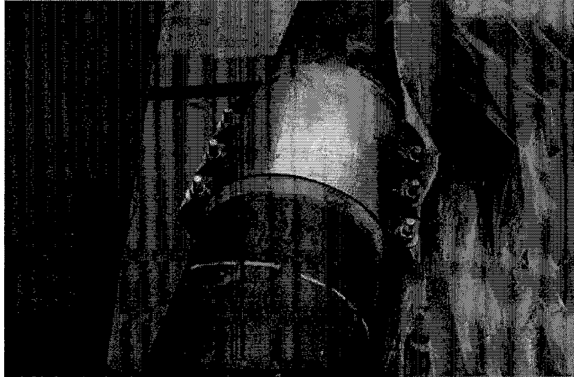
Figure 2 Stainless steel clamp used in conjunction with APPW
