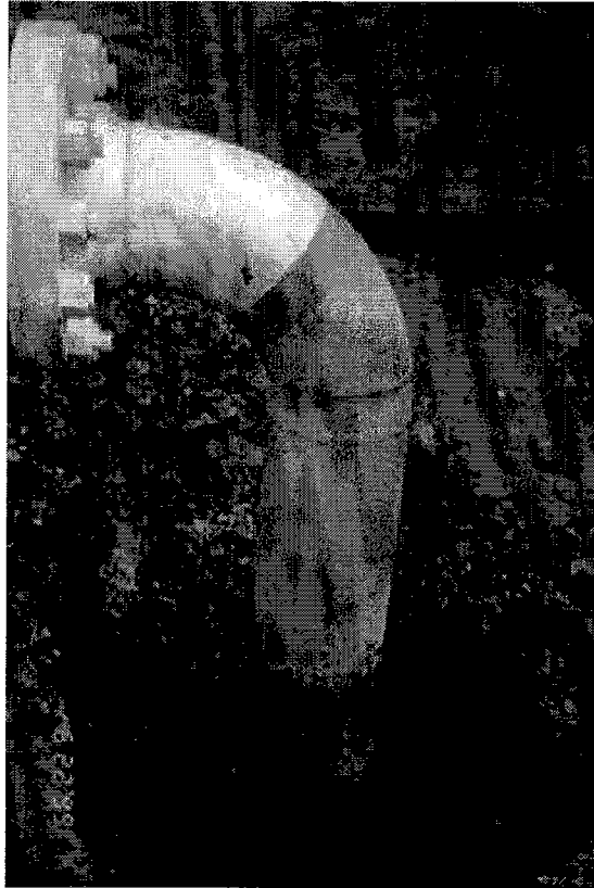
Figure 4 Repair of riser pipe using APPW
