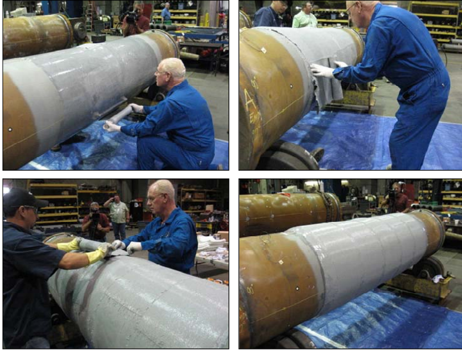
Figure 8 – Photographs showing installation of composite materials on wrinkle bend samples
