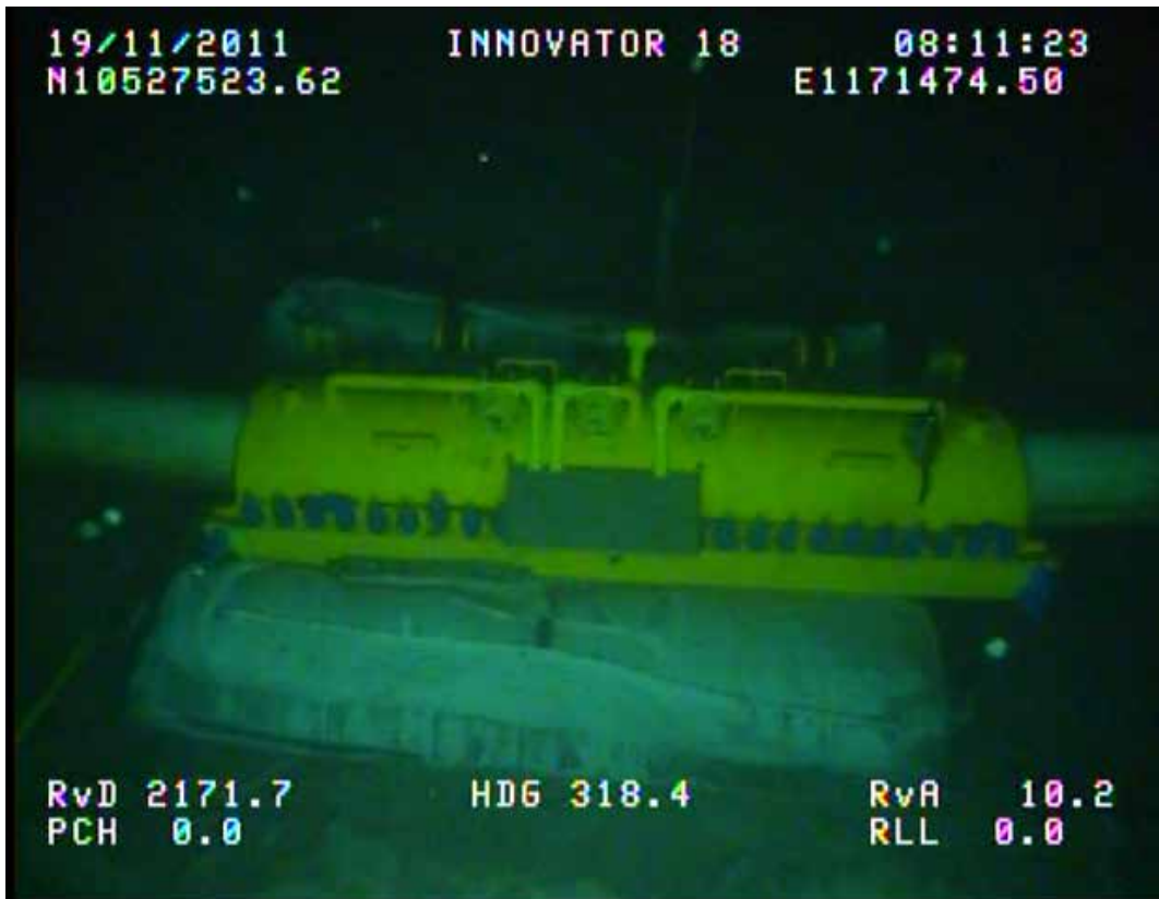
Figure 10 – Grout Sleeve and Grout Bag installed on the pipeline
