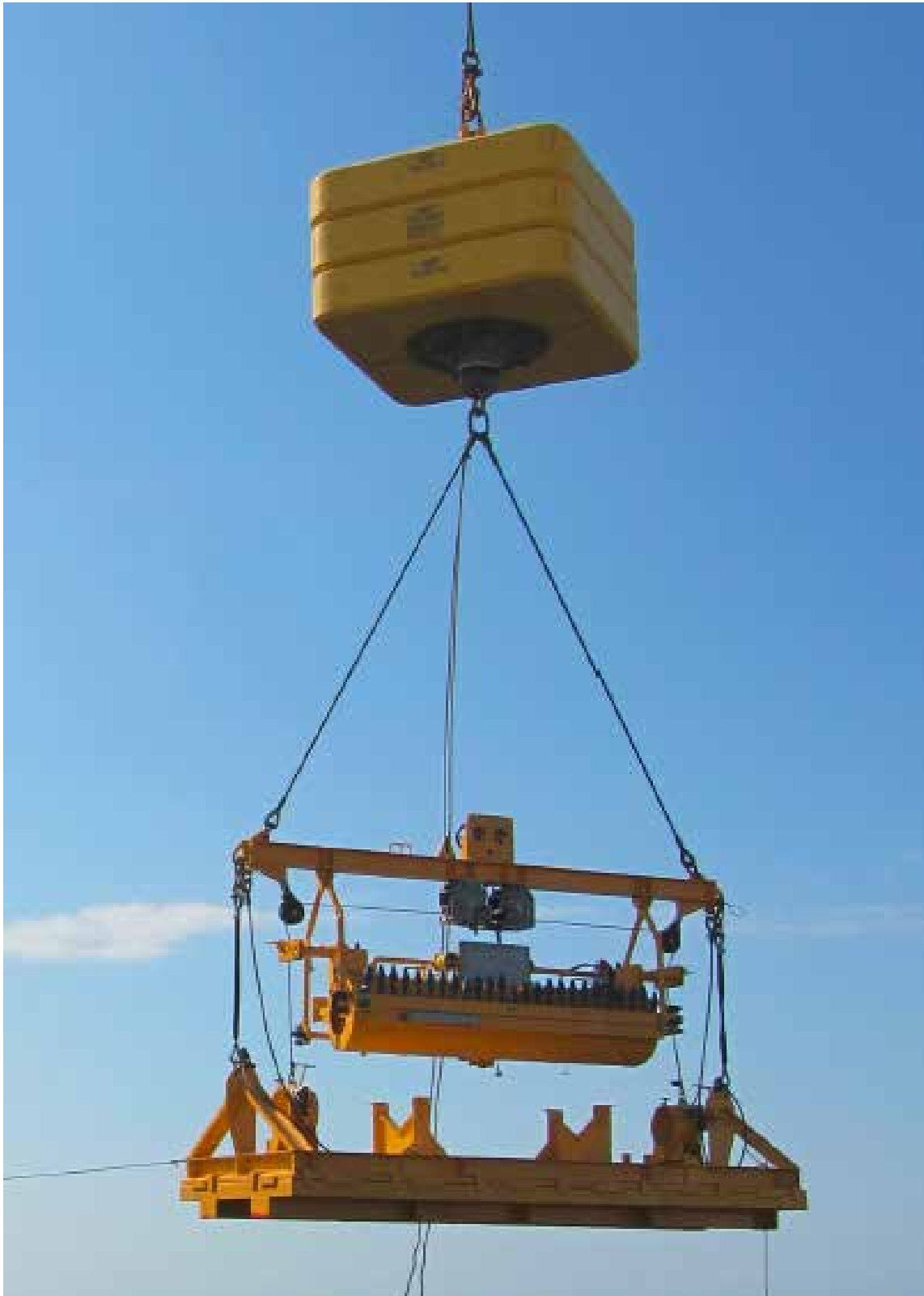
Figure 4 – Grout Sleeve – Suppressor Skid – Buoyancy Module rigged for deployment
