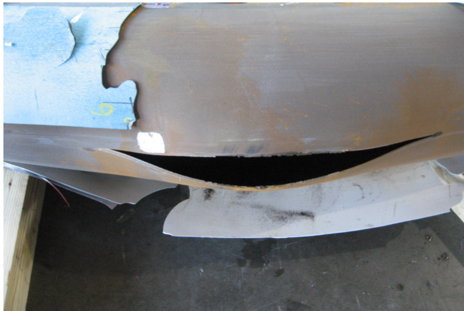
Figure 12 – Close-up photograph of burst failure
