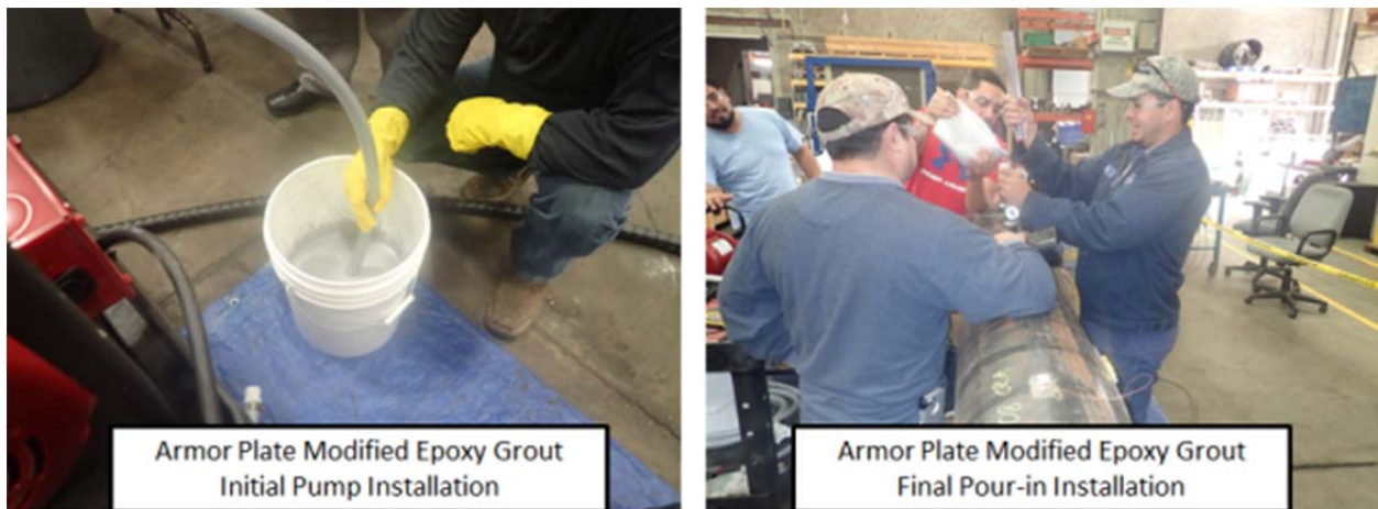
Figure 10: Dent #4, Armor Plate Modified Mix Ratio Epoxy Grout Installation
