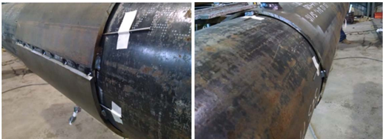
Figure 6: Type B Sleeve Installation
