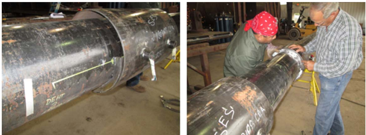
Figure 5: Stand-Off Sleeve Installation
