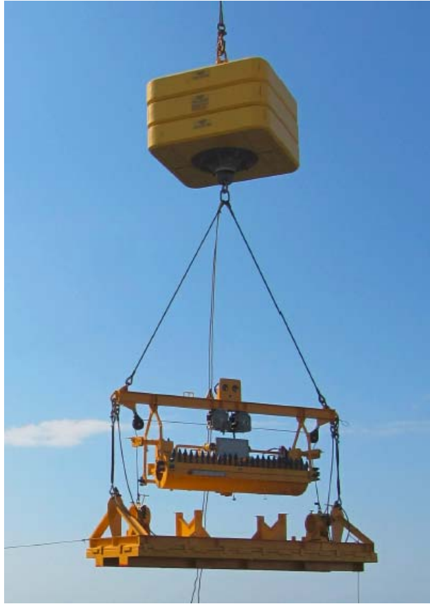
Figure 12 – Grouted sleeve with suppressor skid and buoyancy module rigged for deployment
