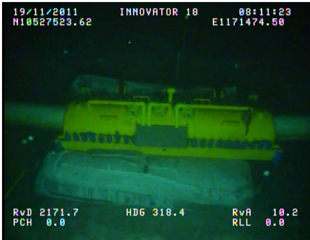
Figure 14 – Grout sleeve and Grout Bag installed on pipeline
