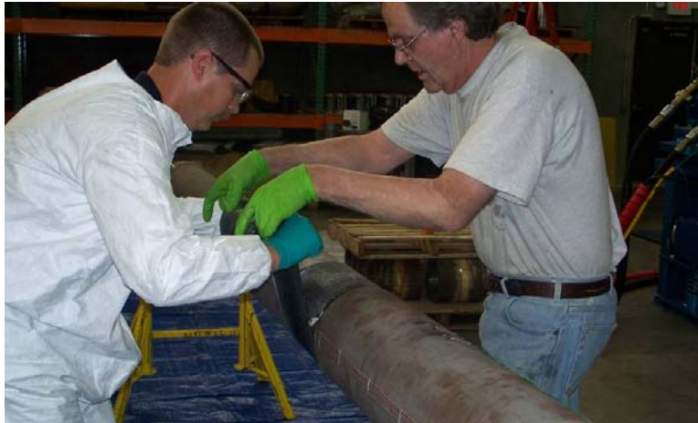
Figure 7 – Installing the hoop wrapped inner carbon layers
