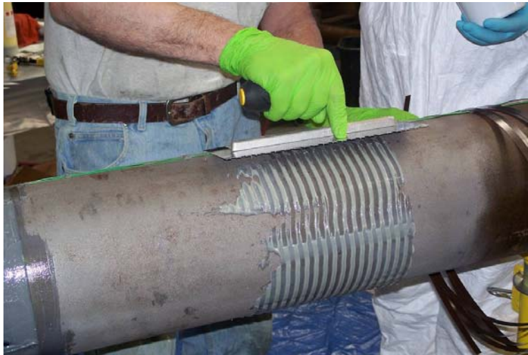
Figure 8 – Applying the epoxy adhesive using a slotted hand trowel
