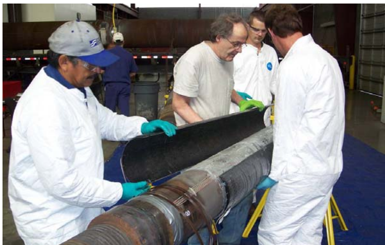
Figure 9 – Installation of the carbon half shells
