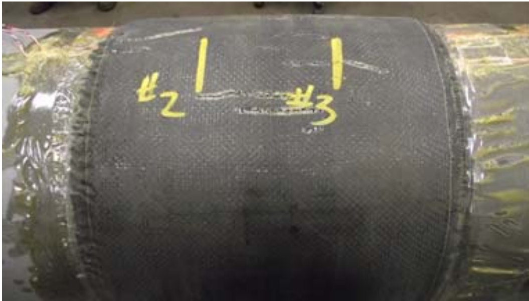
Figure 10 – Photograph of composite repair after installation
