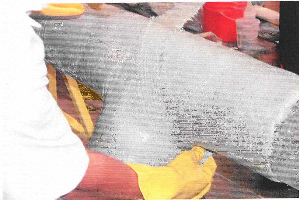
Figure 6 Installation of APPW 360 in a criss-cross pattern on tee
