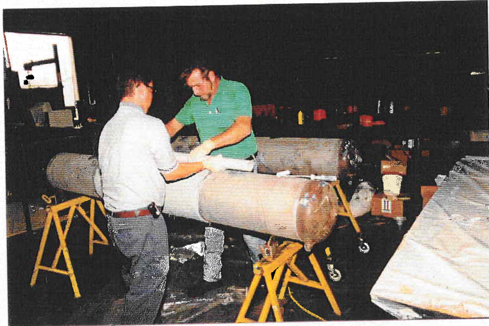
Figure 1 Installation of Armor Plate Pipe Wrap
