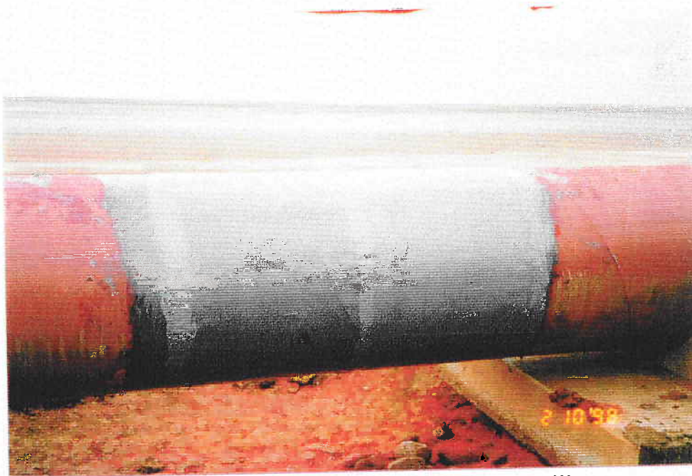
Figure 2 Completed installation of Armor Plate Pipe Wrap
