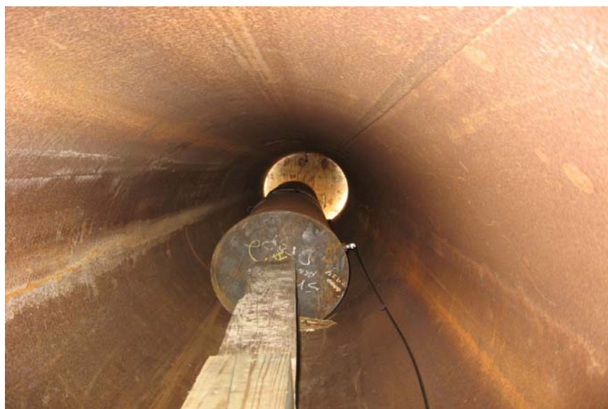
Figure 4 – Sample in Enclosure
