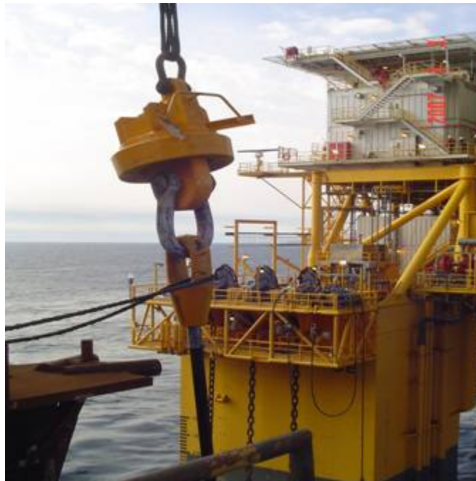
Figure 10 – Cross Haul Bucket during SCR Installation
