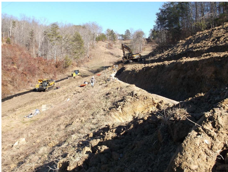
Figure 8: Excavation of pipeline in preparation for installation of monitoring devices (Case Study #3)
