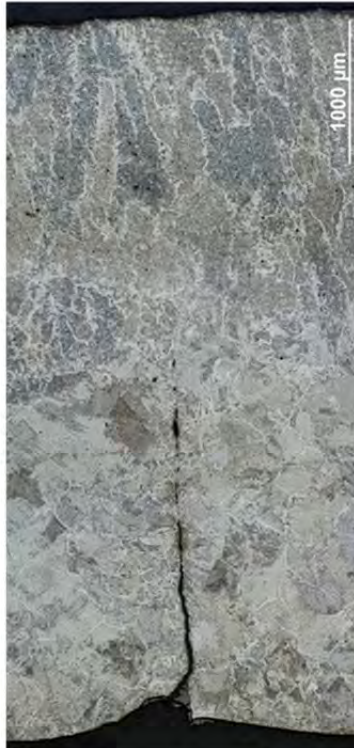
Figure 12: Schematic and photograph showing MATR-3-7 defective girth weld samples
